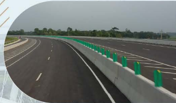
Bridge approach road
