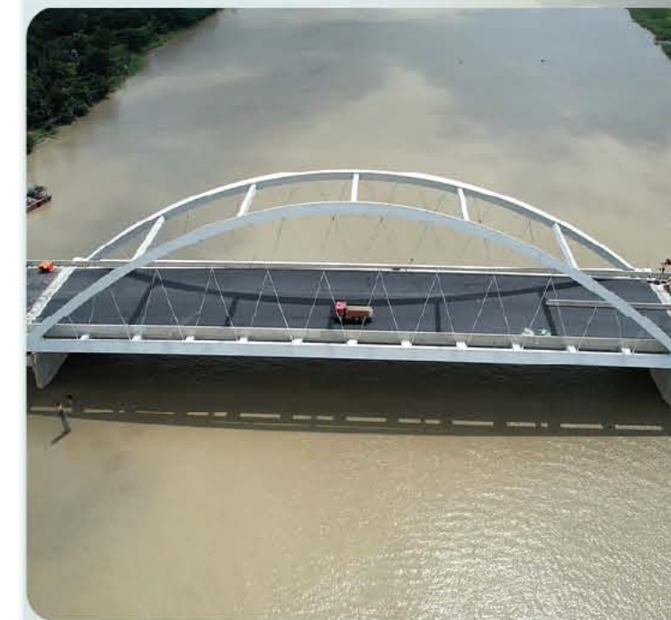
Special arch span of bridge
