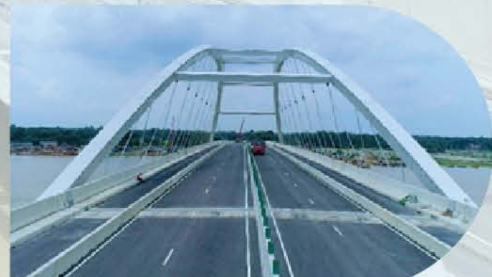
Bridge Center Span
