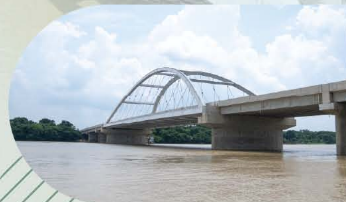
Bridge Side view
